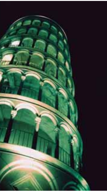
Above Concealed floodlights at each level enhance the texture of the columns and arches.
